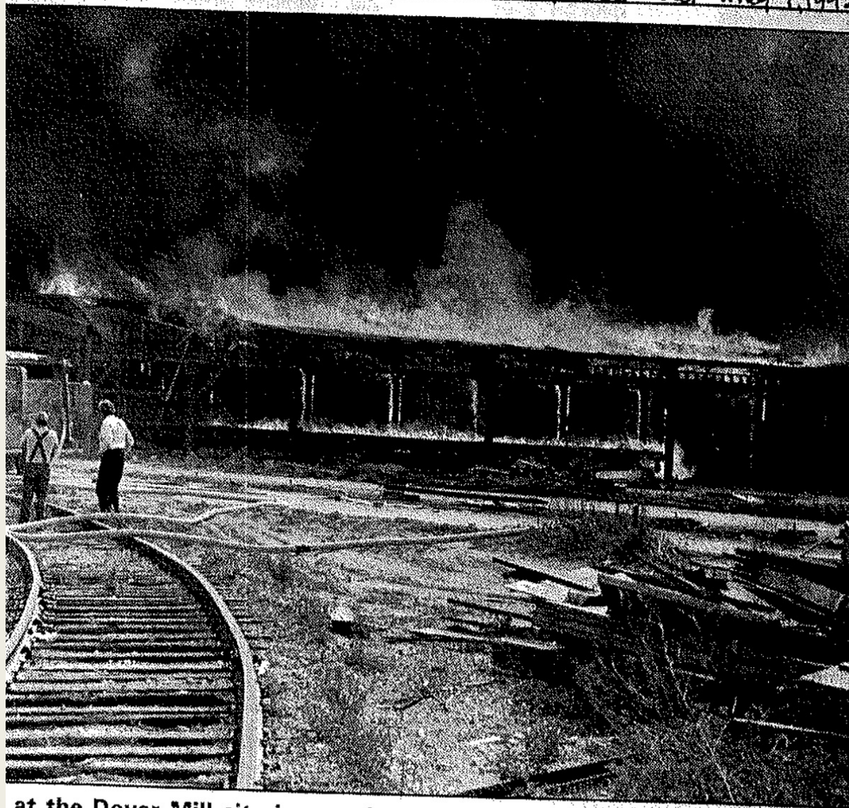
at the Dover Mill site is completely engulfed as firefighters set up their ene.
